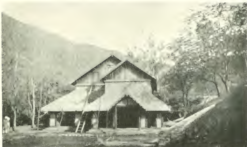
REST-HOUSE AT DULAI; CALLED "HONEYMOON COTTAGE"
